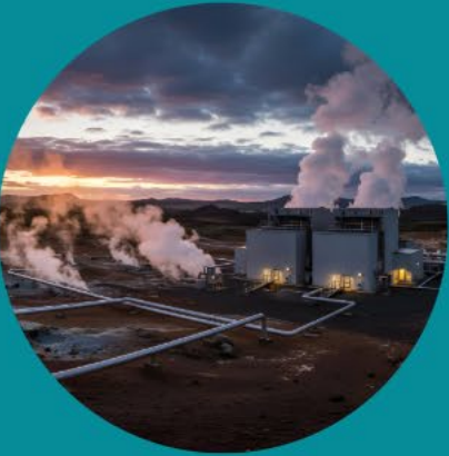
Call Module 06: Heating and cooling technologies
